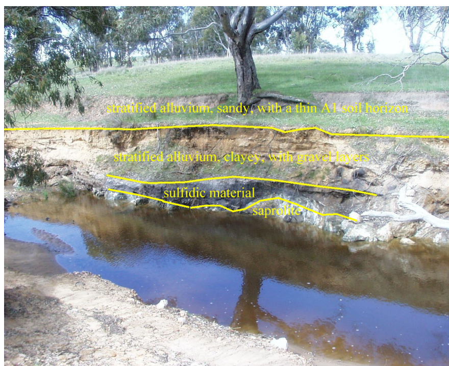
Figure 4.30. An exposure of black sulfidic material in buried acid sulfate soil in a bank section in Dairy Creek. The regolith sequence comprises relatively young sandy alluvium (with a thin soil horizon) overlying older relatively-clay-rich alluvium with thin gravel layers, which may contain fragments of bright yellow oxidised sulfidic materials containing sideronatrite and jarosite (pH <3.5). The sulfuric horizon overlies the black sulfidic materials and saprolite (derived from Tapanappa Formation lithologies). Note the white salt efflorescences (halite, gypsum) just above the water line.
